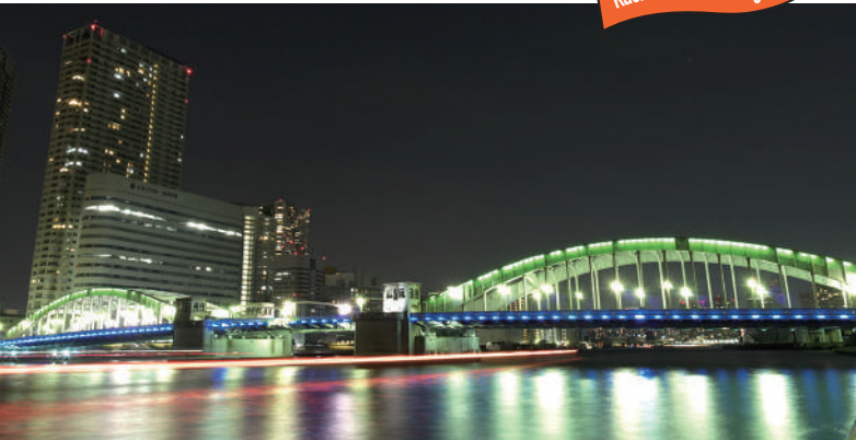
The two ends of the bridge are arches, while the center was built as a drawbridge opening upward in the center (though it currently does not open)
